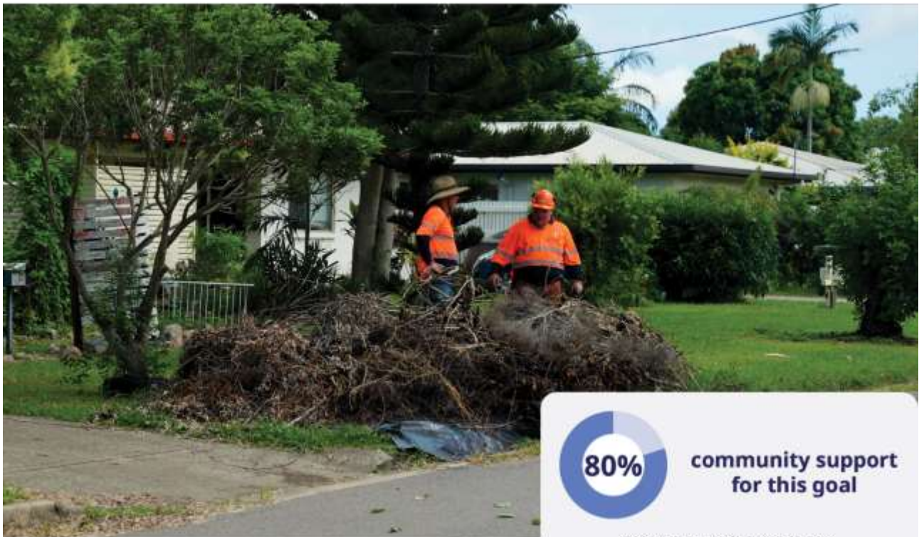
Tropical Cyclone Kirrily clean up
